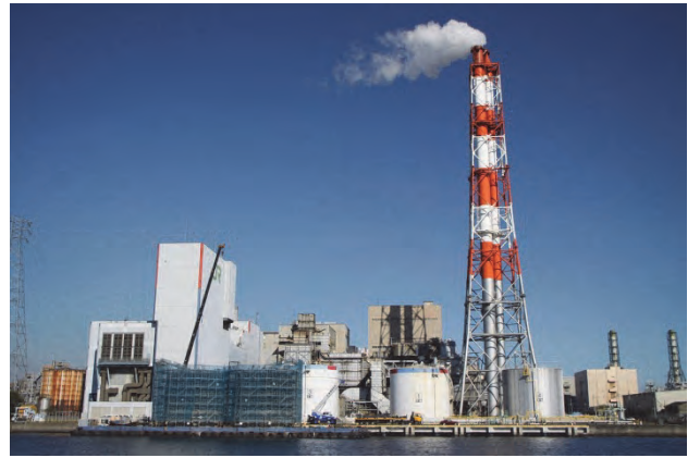
Kawasaki thermal power plant
